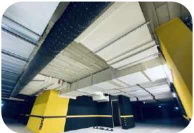
Combination of ventilation and smoke extraction ducts saves space
