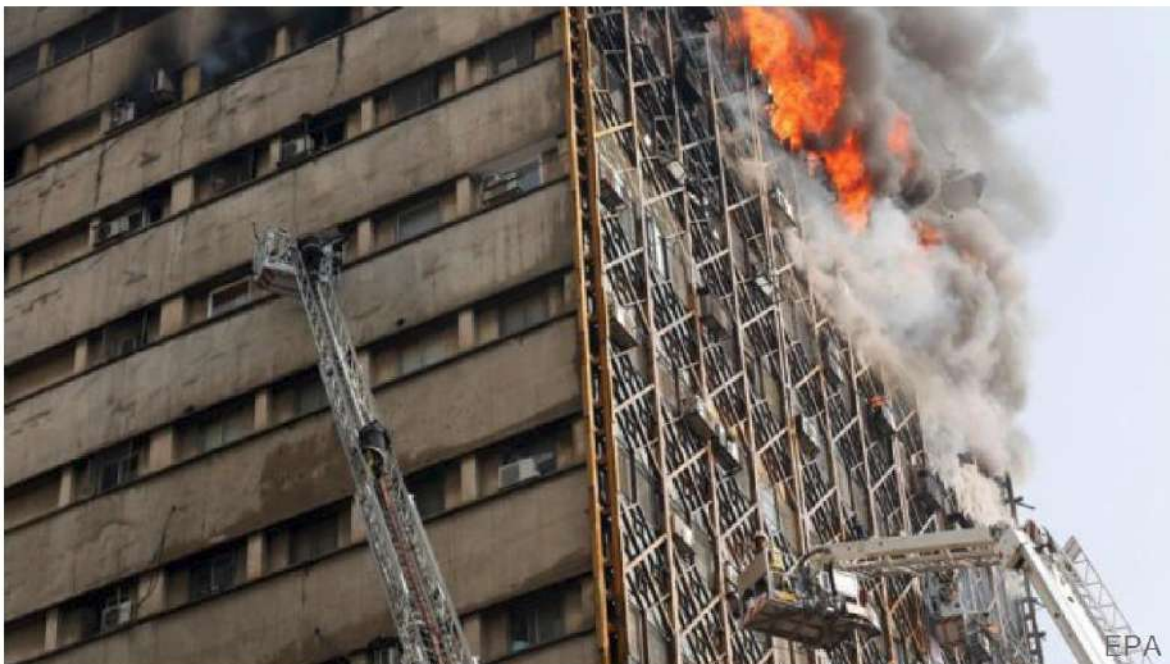
Firefighters battled the blaze for hours before the block collapsed
